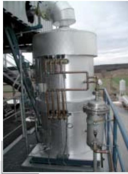
Photo of the catalytic tar reformer at the biomass power plant in Güssing, Austria and a detailed view
